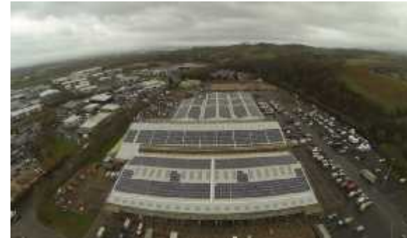
Solar panel array on the Livestock Centre
