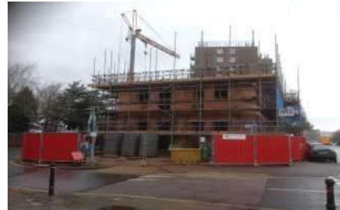
Work in progress at Vaughan Road
