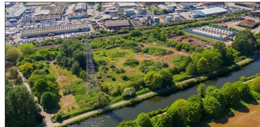
Solar farm and storage project
