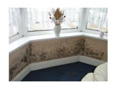
**Condensation dampness** occurs when warm, moist air inside a dwelling meets a cold surface (such as an external wall or the inside surface of a cupboard). The air cools at the contact point and the moisture in the air becomes a liquid. The colder the surface, the greater the likelihood of condensation. The moisture left on surfaces as a result of condensation will encourage mould growth.
