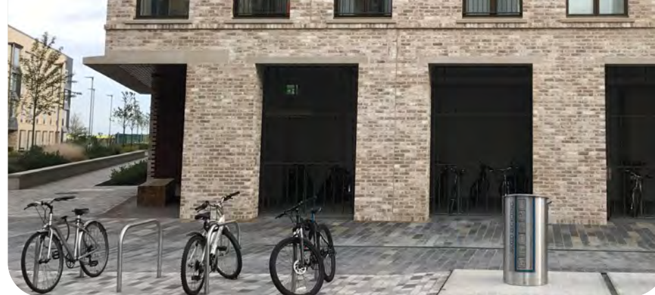
Convenient and secure visitor and resident cycle parking both on street and within buildings, Cambridge
