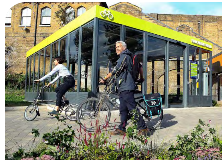
Cycle hub with attractive and secure cycle parking. © Copyright 2018 Enfield Council
