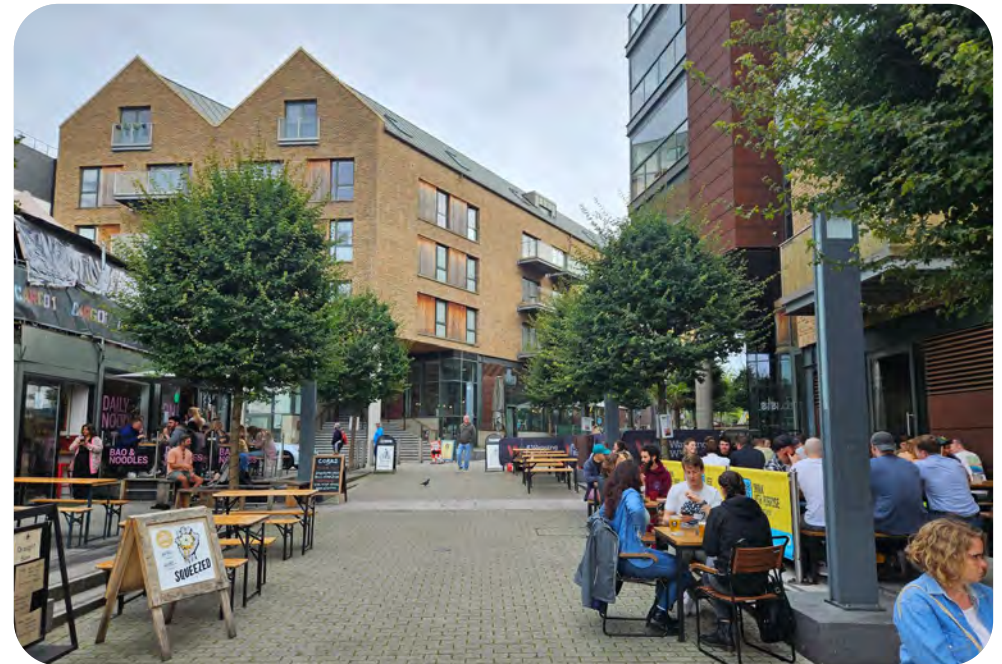
Wapping Wharf Phase 1 Mixed-use scheme, which integrates new flats and ground floor retail space along Bristol Harbour.
