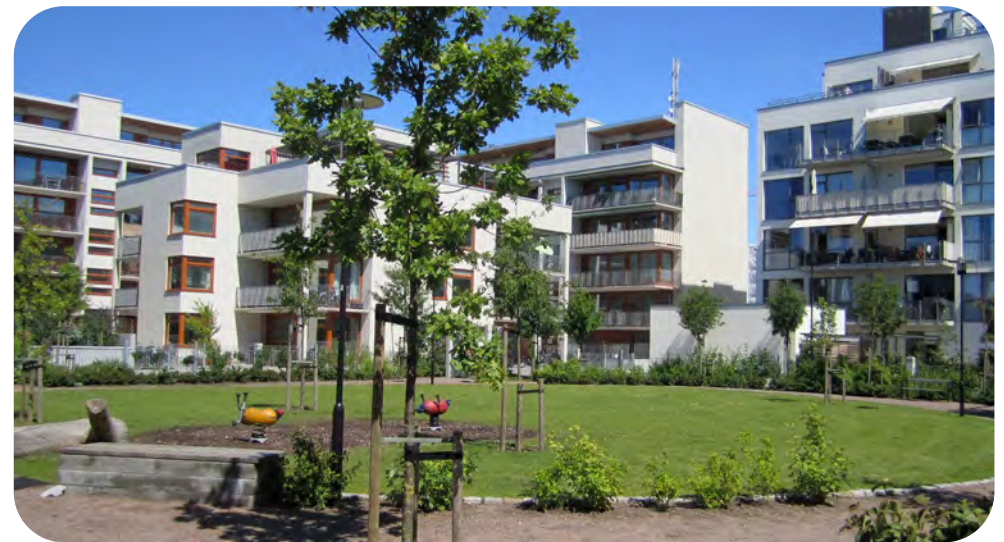
Apartment blocks which cater for a broad demographic including families with easy access to play and open space, Malmo, Sweden
