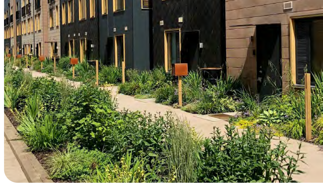
Raingardens incorporated within streets and hard impermeable surfacing kept to a minimum, Leeds Climate Innovation District.
