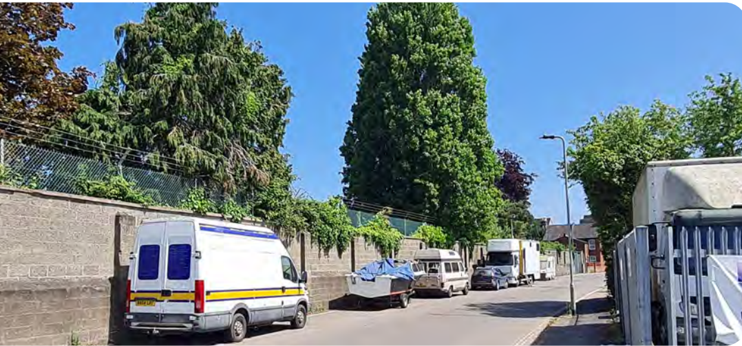
View of Water Lane showing the relatively narrow existing street width and significant height difference behind the retaining wall to the north.
