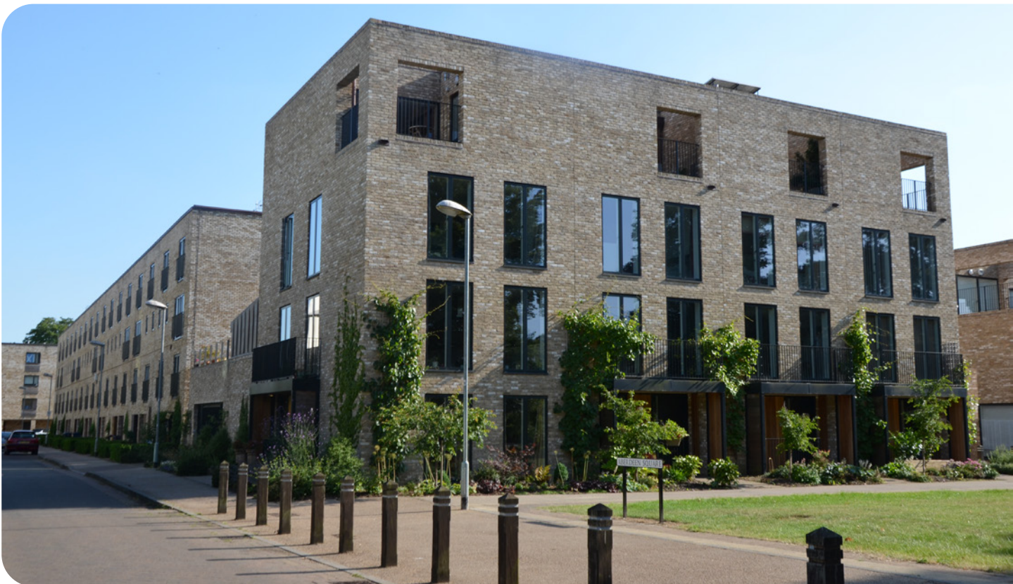
High-quality homes with dual aspect dwellings and great access to both private and communal outdoor space, Accordia, Cambridge
