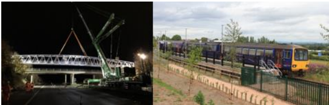
Recent Projects, Tithebarn Pedestrian/Cycle Bridge and Newcourt Railway Station
