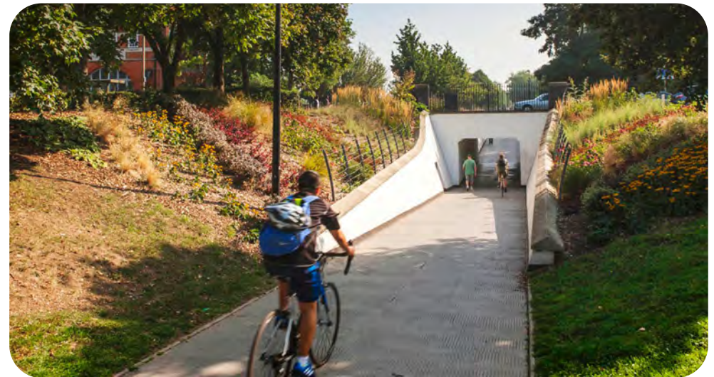
Underpass with good sightlines and daylight, Burgess Park, London. Image credit, Robin Forster Photography.
