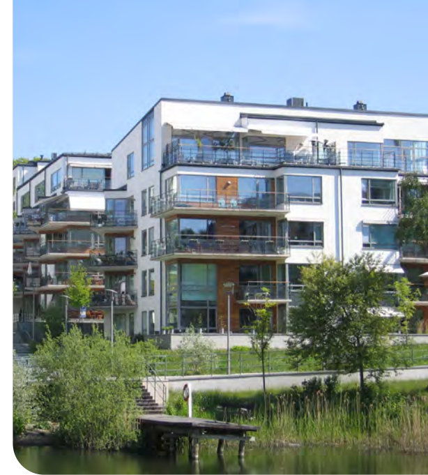
Positive interface with the water, and well considered setback incorporating mature trees at Hammarby Sjostad, Sweden.
