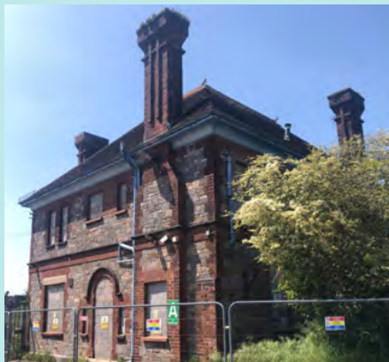
Gas Works former Social Club
