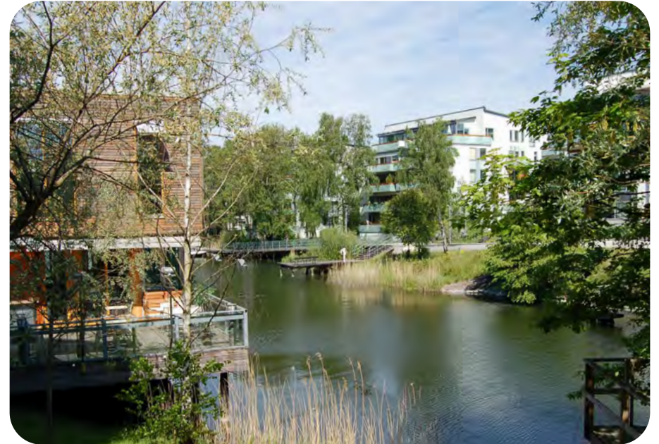
Integrated energy, water and waste resource strategies embedded into Hammarby Sjöstad, Sweden
